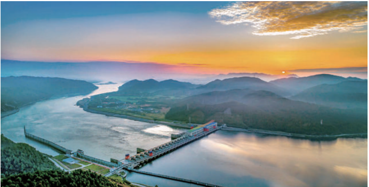
中国中铁在鄱阳湖生态经济区建设的重点水利工程——峡江水利枢纽工程 Xijiang water conservancy hub project - the key water conservancy project built by CREC in Poyang Lake's ecological and economic zone
