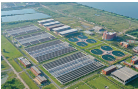
● 中国中铁建设的国内一次性建成规模最大的污水处理厂——武汉北湖污水处理厂项目 Wuhan Beihu Wastewater Treatment Plant – the largest domestic sewage treatment plant built by CREC at one time
