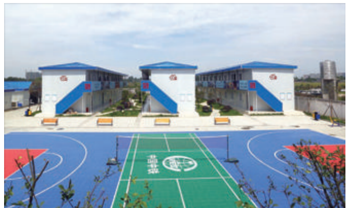
● 中国中铁广泛开展工地“幸福之家”建设 CREC extensively carried out the construction of "happy family" projects at construction sites
