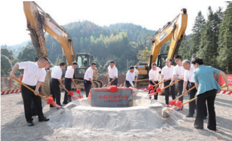
中国中铁在湖南省桂东县捐建的中铁振兴大道正式开工 The CREC Revitalization Avenue in Guidong County, Hunan Province donated by China Railway was officially commenced
